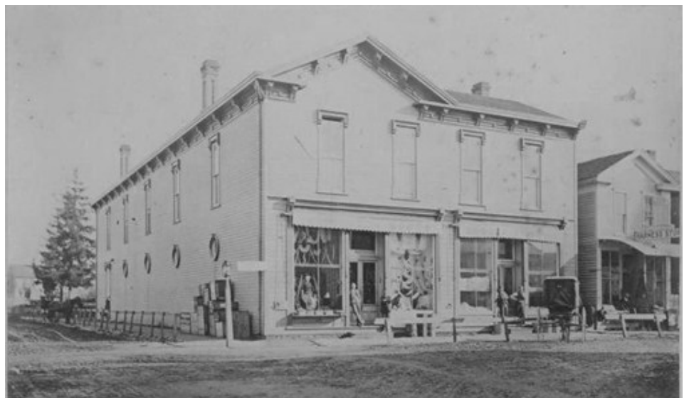
Poorman's Dry Goods Store located in St. Paris.
